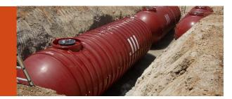
Vapor monitoring measures either product vapors in the soil around the UST, referred to as passive monitoring, or special tracer chemicals added to the UST, referred to as active monitoring.
