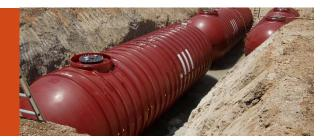
Secondary containment uses a barrier, an outer wall, or a liner around the UST or piping to provide secondary containment. Tanks can also be equipped with inner bladders that provide secondary containment.
