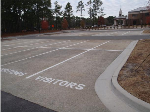
**Figure 12. Pervious Concrete Parking Stalls.**
