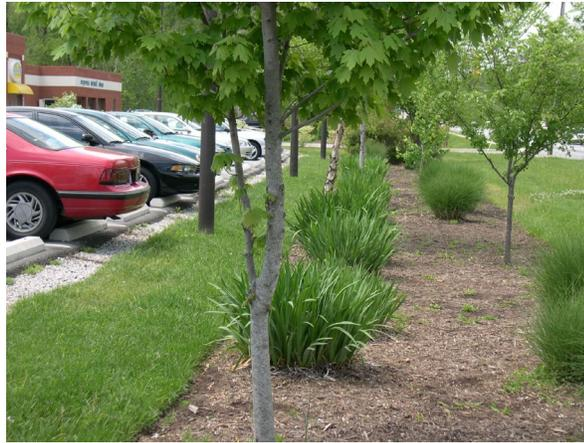
**Figure 8. Bioretention Incorporated into Traditional Parking Lot Design.**
