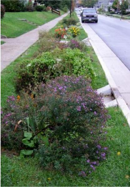
**Figure 7. Bioretention Incorporated into a Right-of-Way.**
