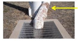
Overflows directly connected to a sanitary sewer or storm drain will trigger a significant deficiency; there must be an air gap of at least 3 pipe diameters above the sanitary sewer or storm drain.
