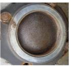
The #24 mesh screen can be used to keep contamination out. The screen should be inspected after overflow events and replaced, if necessary.
