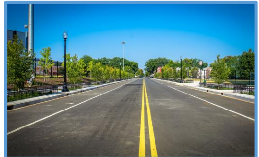
O Street NW is lined with rain gardens, sidewalk trees and other green features.
