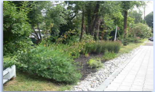
Rain Garden in Forest Heights, Maryland
