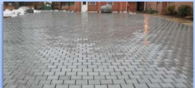
Permeable pavement in Forest Heights, Maryland
