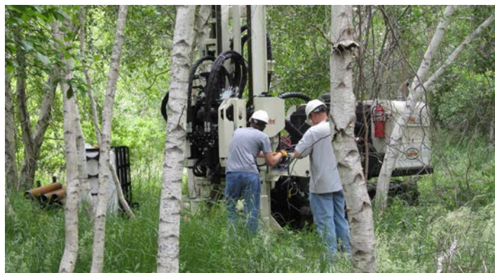
GWERC scientists installing monitoring wells in Rhode Island
