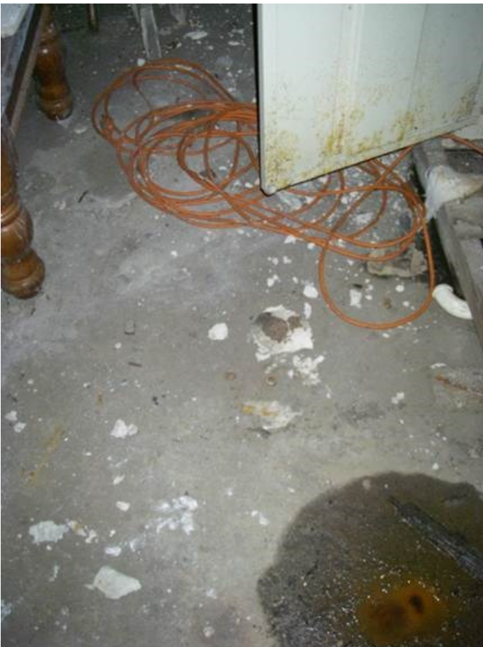
Regulated asbestos-containing material on floor.
