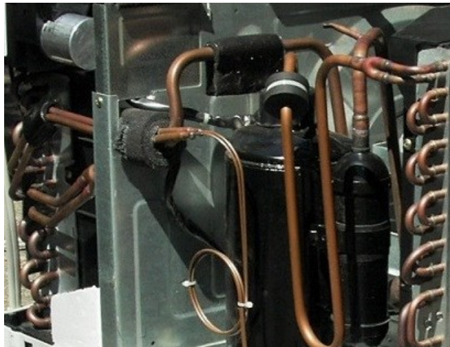
Copper tubing in air conditioning unit (stock photo)
