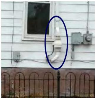
Vapor mitigation system installed on the outside of a house.
