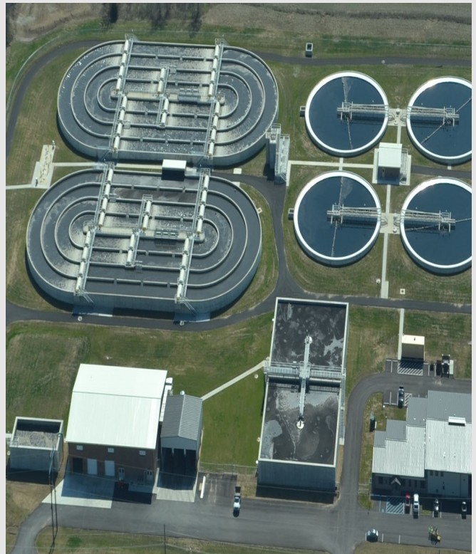
New wastewater treatment plant in Columbus, Indiana
