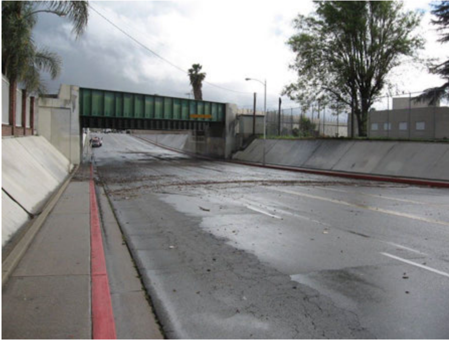
Photograph 2: View of railroad bridge and pump station, camera facing southeast, May 23, 2016
