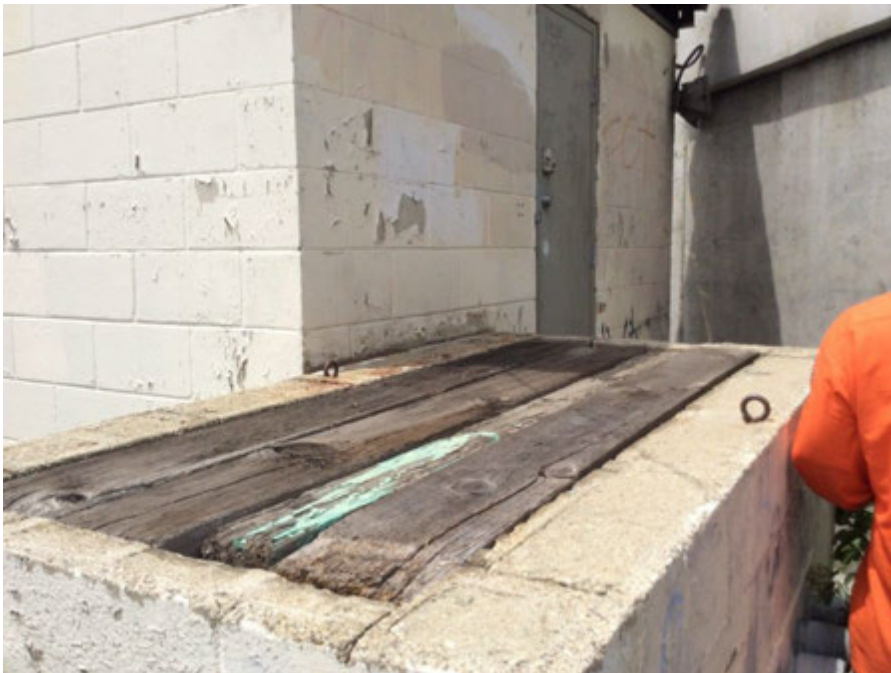
Photograph 3: View of south elevation of pump station, camera facing east, May 23, 2016
