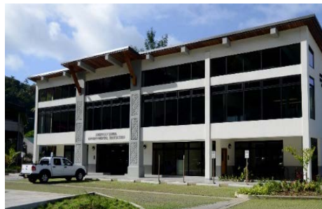
Left: The Agingan Wastewater Treatment Plant in Saipan, Commonwealth of the Northern Mariana Islands. (EPA OIG photo)
