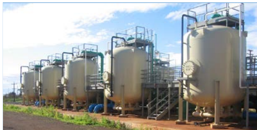
The Ewa Shaft Granular Activated Carbon Treatment Facility, on Hawaii's island of Oahu, received Drinking Water State Revolving Funds. (Hawaii Department of Health photo)
