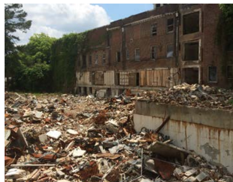
Exposed debris potentially including significant asbestos-containing material at the Old Davis Hospital in Statesville, North Carolina. (EPA photo)
