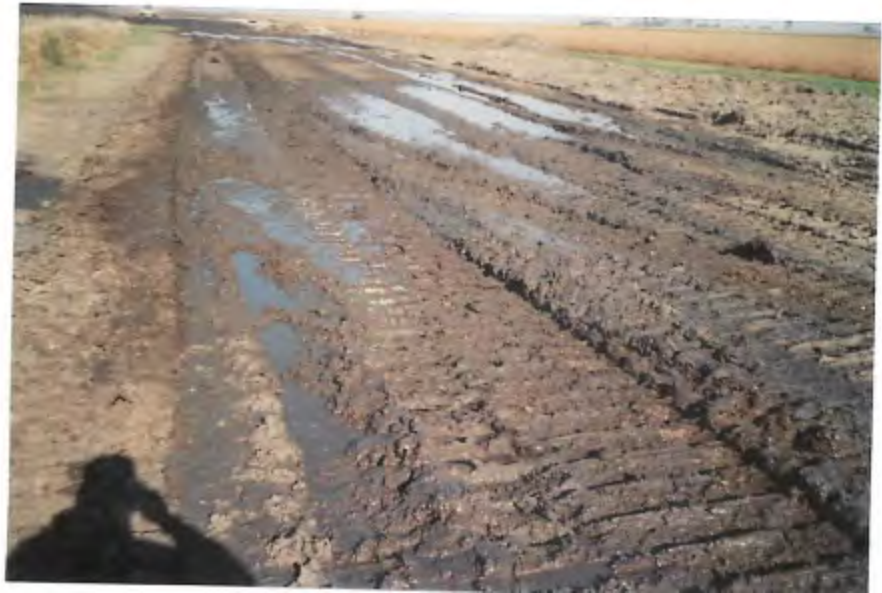
Figure 4: Unnamed farm in northern LaSalle County. Subsoil layers and topsoil intermixed on replacement. No tile or tile damaged and not functioning
