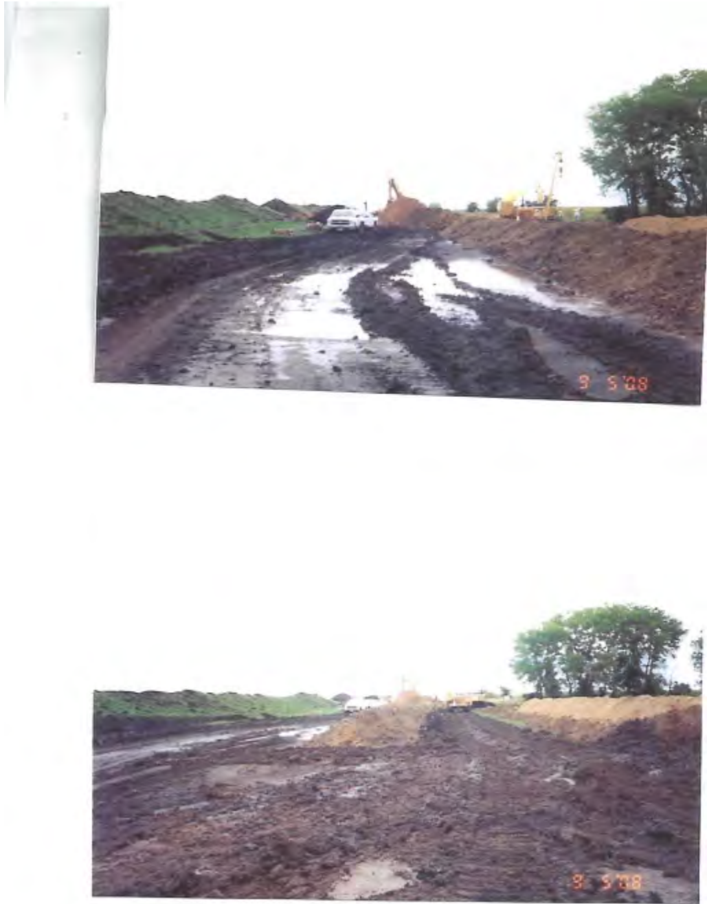
Figure 5: working in wet, saturated soil conditions. Note the 2 piles of subsoil
