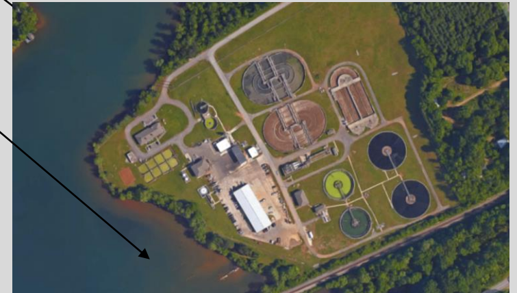
Concord wastewater treatment plant
