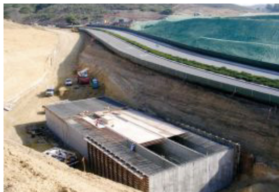
Located just uphill of the resort's grand-entrance bridge, the water quality system's largest cistern holds 540,000 gallons of water.
