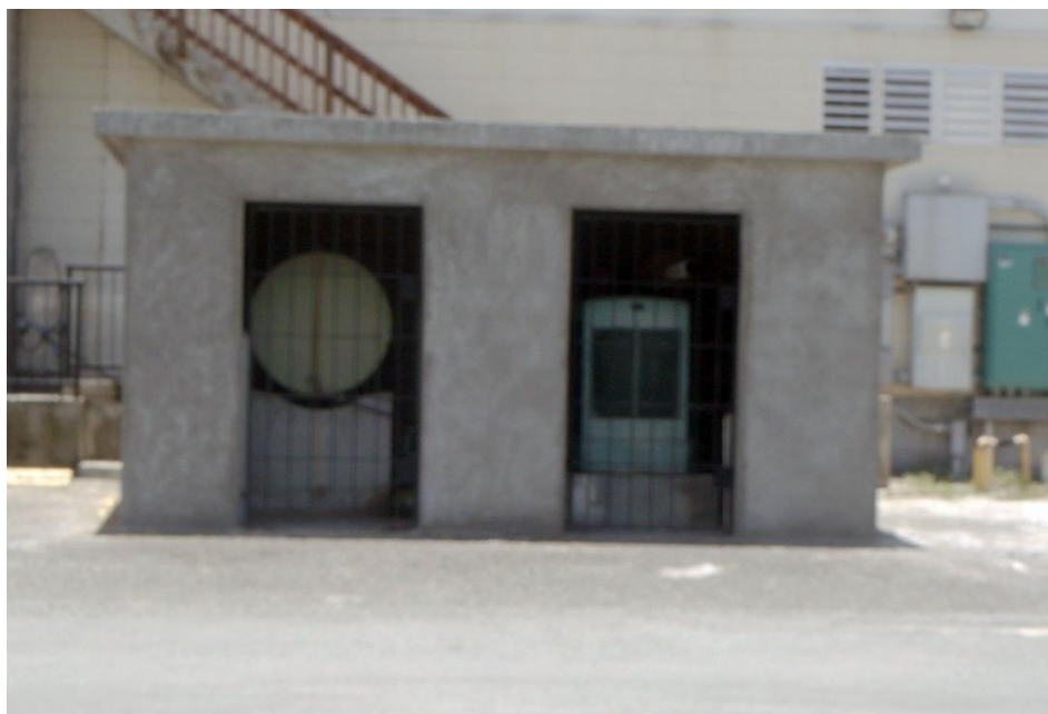
Figure IV.C.21. Diesel tank without containment adjacent to well.
