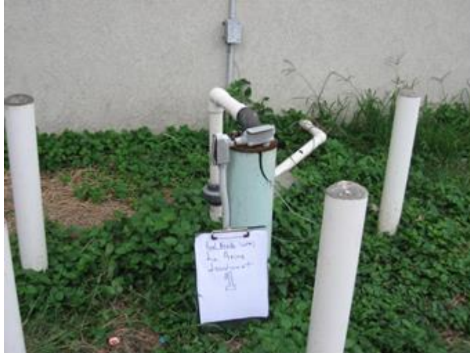
The initial inspection well has no meter.
