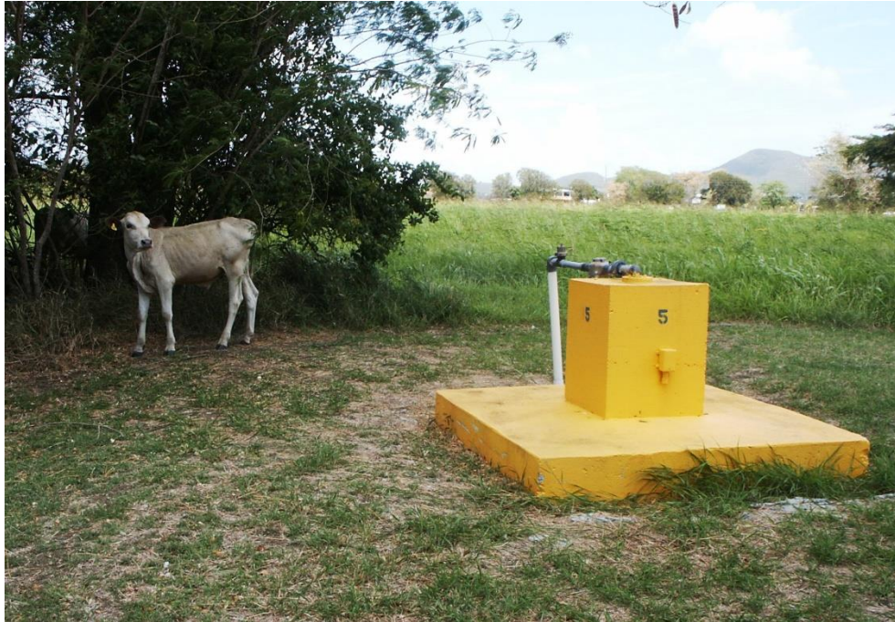
Figure IV.C.10. WAPA well with typical platform and riser.
