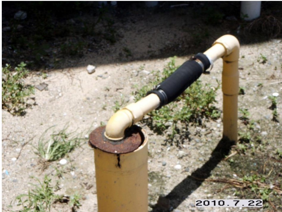
Figure IV.C.20. Laundromat well without effective seal.
