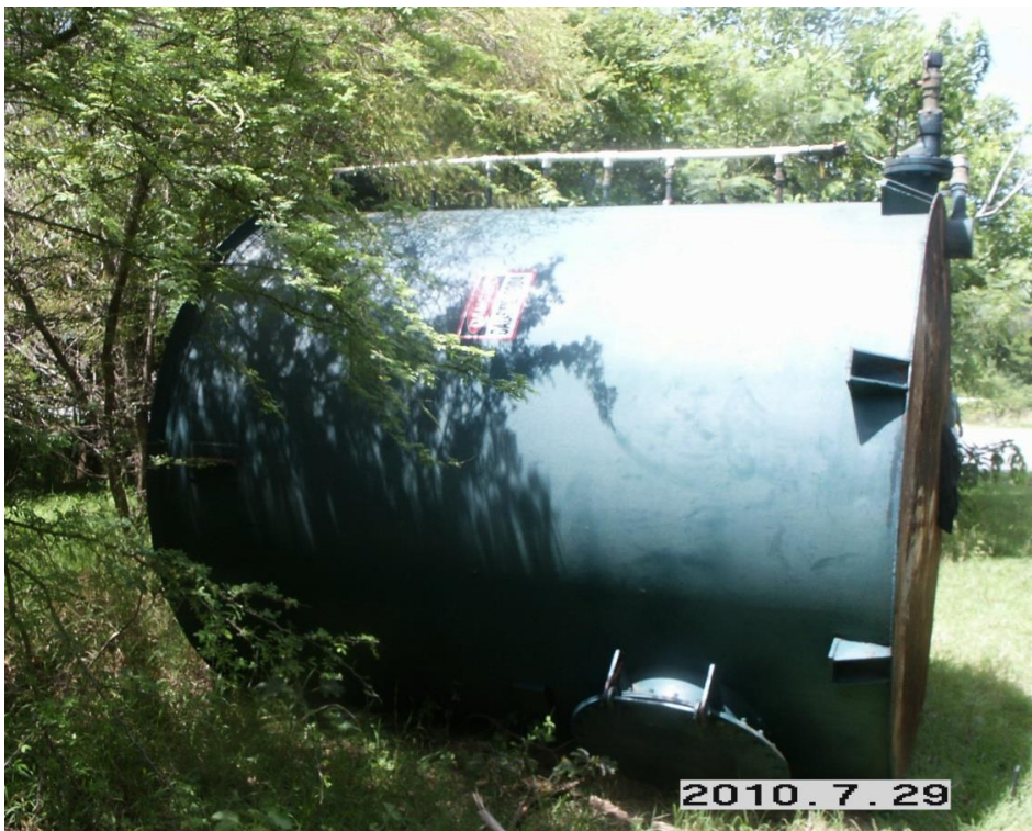
Figure IV.C.25. Abandoned Caustic tank near Bethlehem Ghut and wells.
