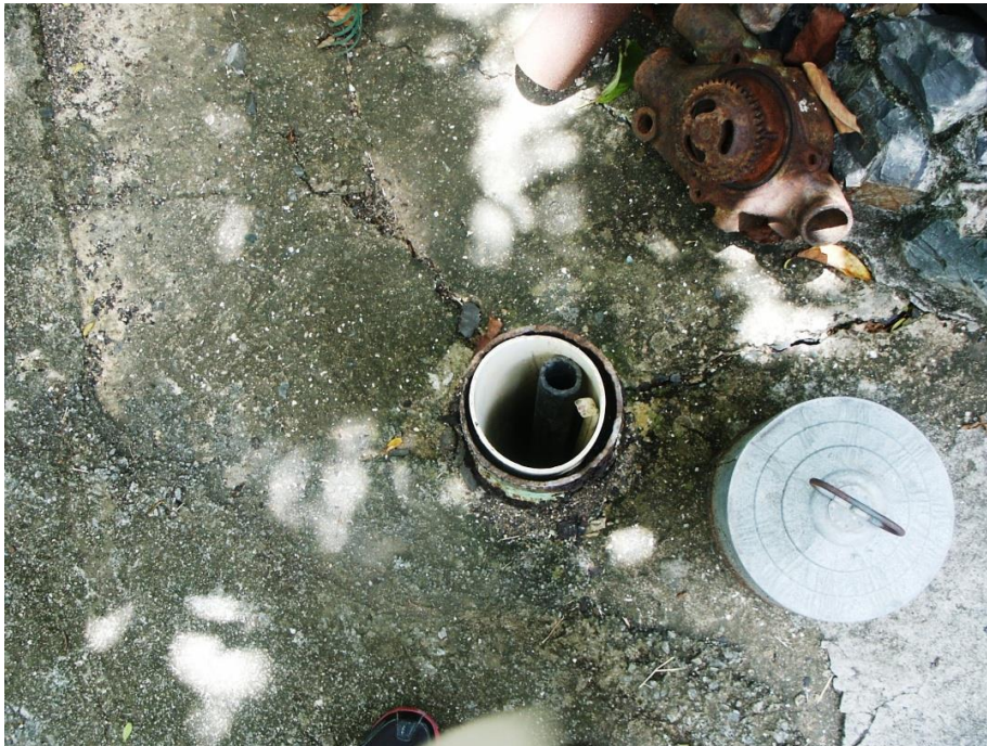
Figure IV.C.23. What's under the cover; this abandoned well is adjacent to a production well providing potable water.
