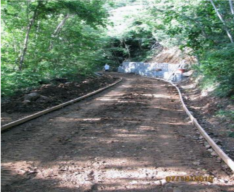
Fish Bay: retaining wall and subdivision road.
