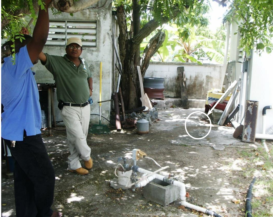
Figure IV.C.22. Production well for vendor; note the galvanvanized cover.
