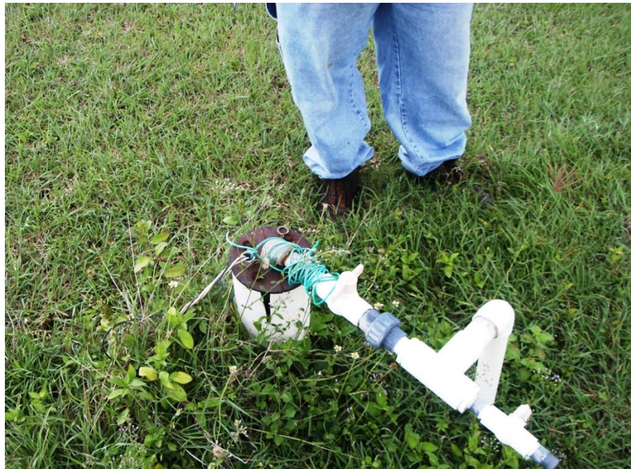
Figure IV.C.15. Wellhead with compromised sanitary seal and cut in casing.
