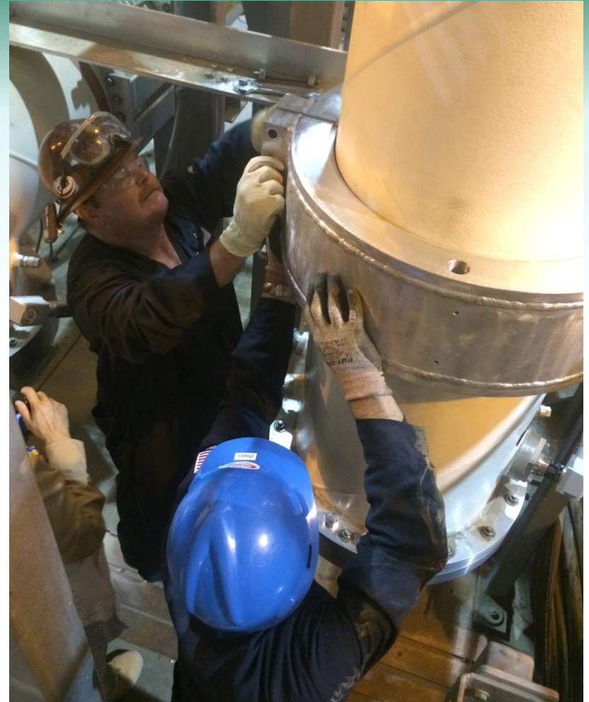
Installation of enclosure
