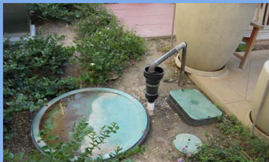
Connection to storage tank
