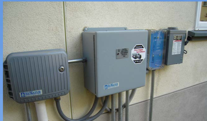
Irrigation And Pump Controllers
