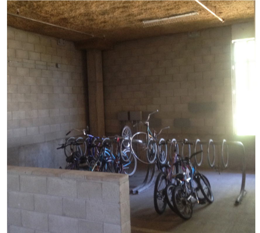
Space for tank?
