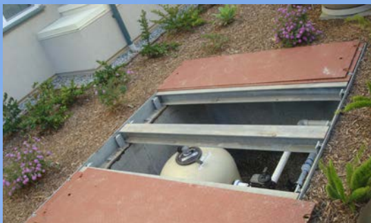
Sand Filter System
