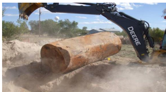
Tank removal at Batesland store (former Mobil Oil and gas station), Pine Ridge Reservation, South Dakota. Batesland is on the national backlog, and the EPA is performing cleanup actions at the site. (EPA photo)
