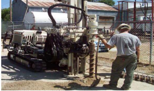
Monitoring well installation, Pine Ridge Oil Company (Pine Ridge Indian Reservation, South Dakota, Oglala Sioux Tribe). During fiscal year 2016, EPA funding was used to remove contamination at two sites. (EPA photo)
