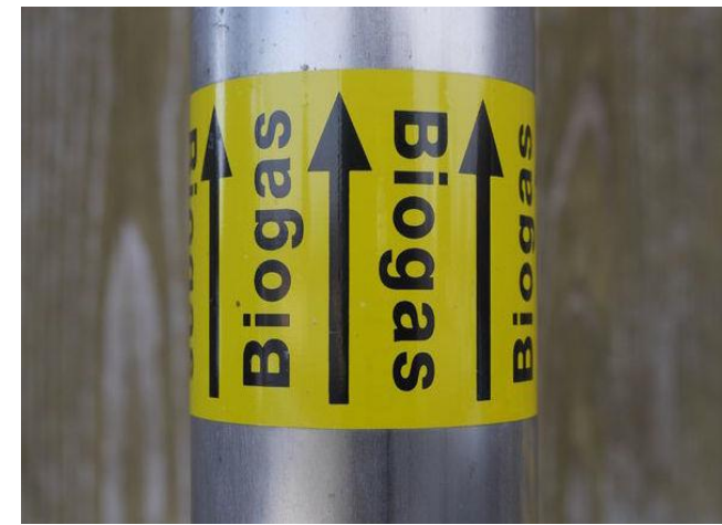
Biogas handling equipment
