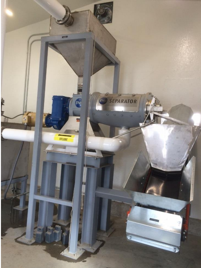
Digestate solids screwpress
