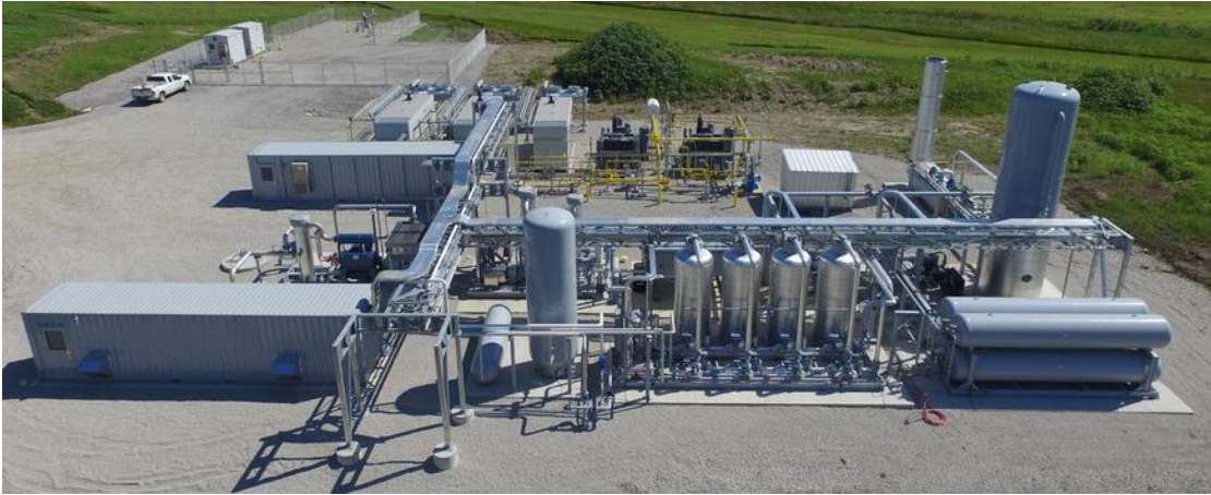
Biogas to pipeline quality biomethane processing facility
