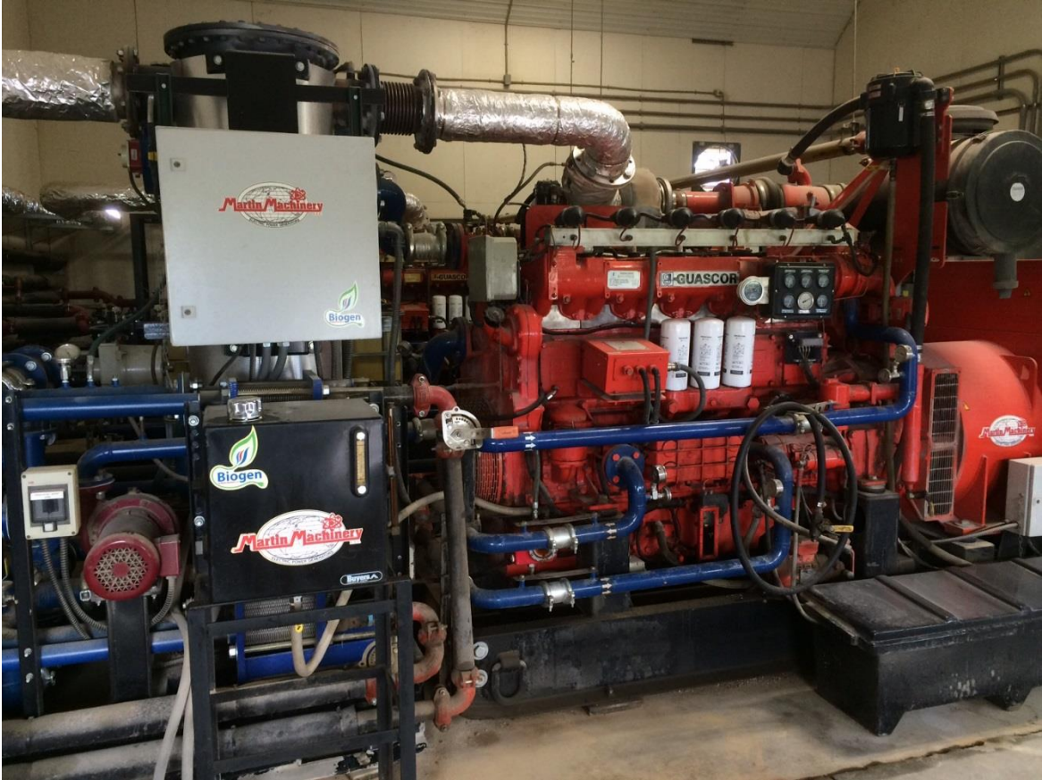
Internal combustion engine for electricity generation
