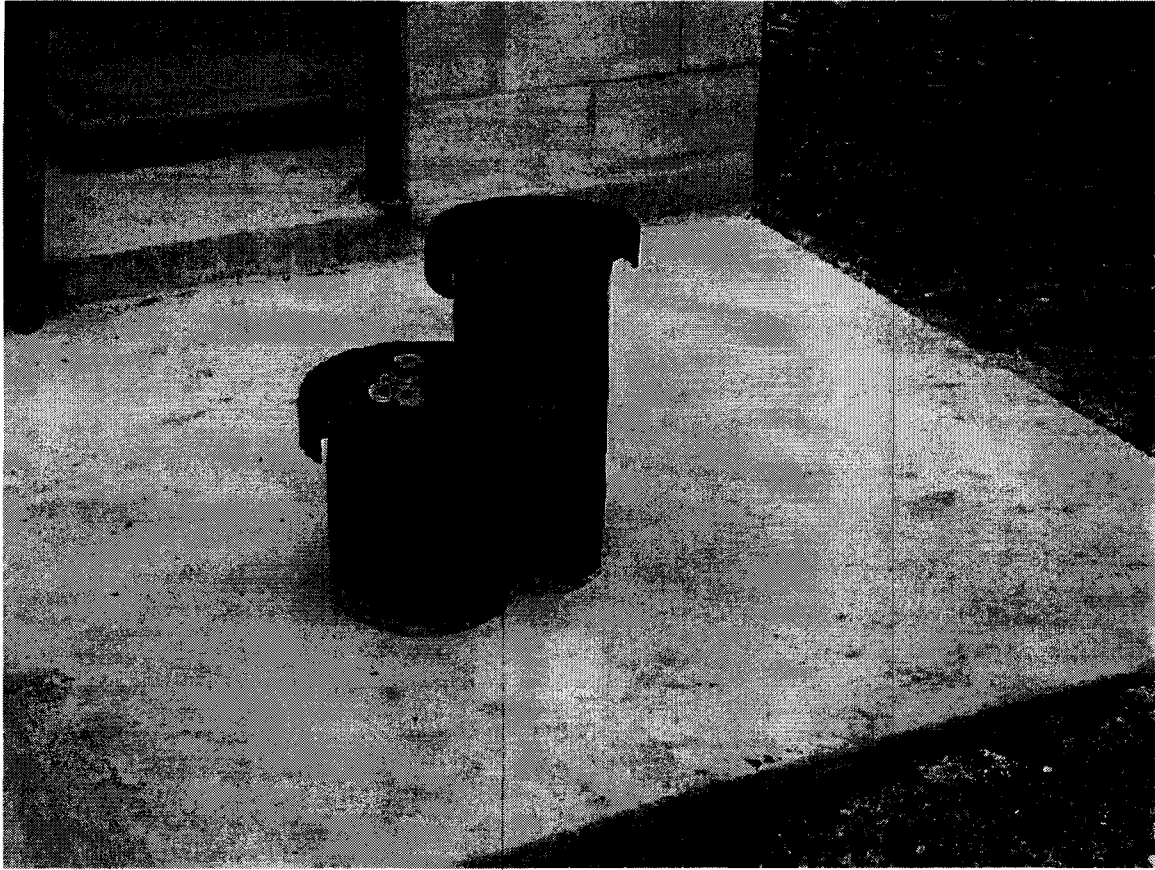
Close-up of the Halawa Deep Monitor Well (2295-03) Picture Shows Well Casing and Housing For Handar Instrumentation
