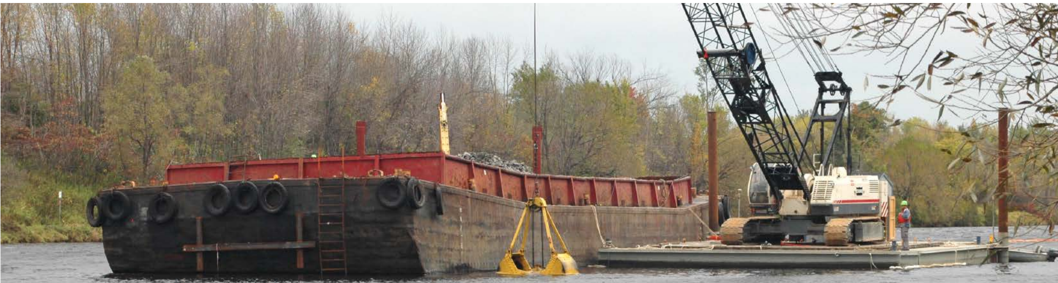
Photo: 2005 Remedial Options Pilot Study – Armor Stone Placement
