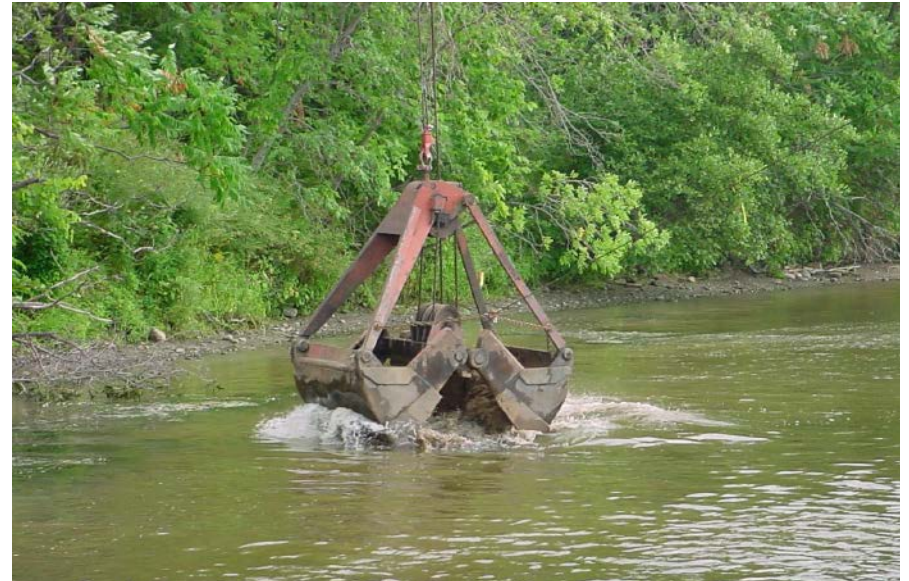
Photo: Capping Pilot Study - Cap Material Placement
