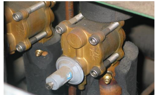
Image of a Schrader valve with no caps
