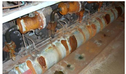
Excessive corrosion on rack components
