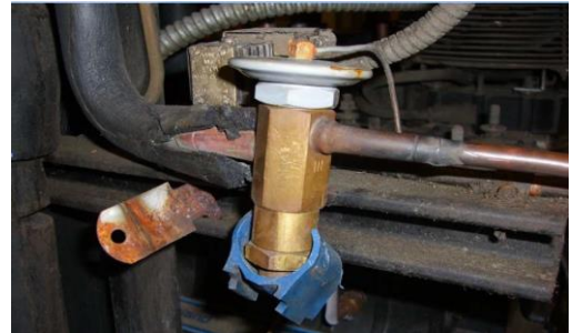
Image of broken clamp caused by vibrations
