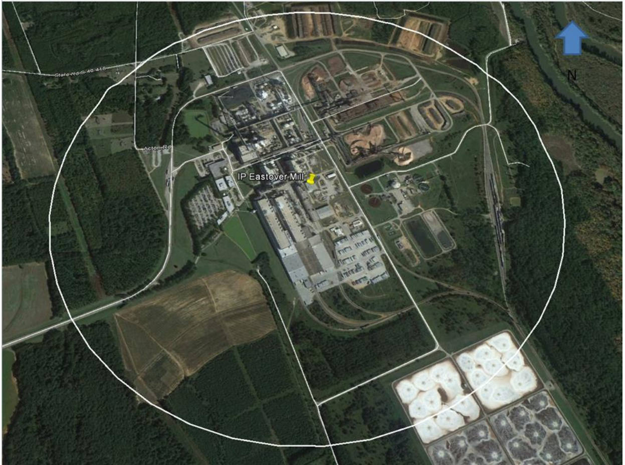
Figure 5 Area surrounding IP Eastover Mill with 1 km radius circle
