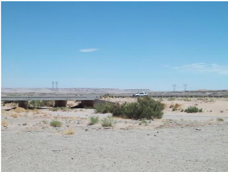
Photo 6: Mine Site #121; Drainage at south end and Hwy 89
