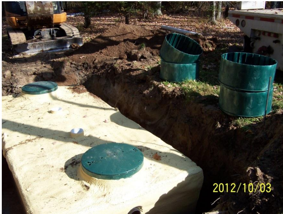
Photo 3. The installation of an insulated holding tank for a seasonal dwelling.
