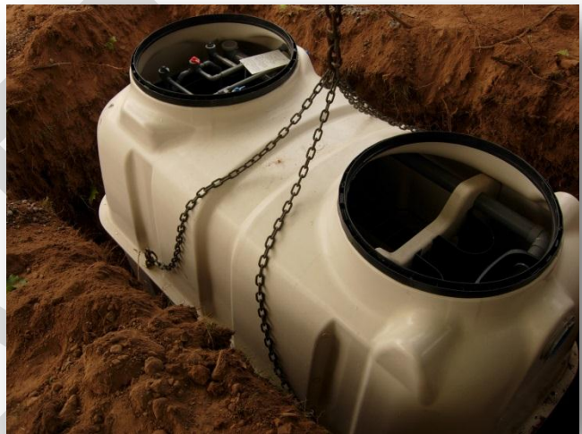
Photo 2. Example of type IV system using a registered treatment product.
