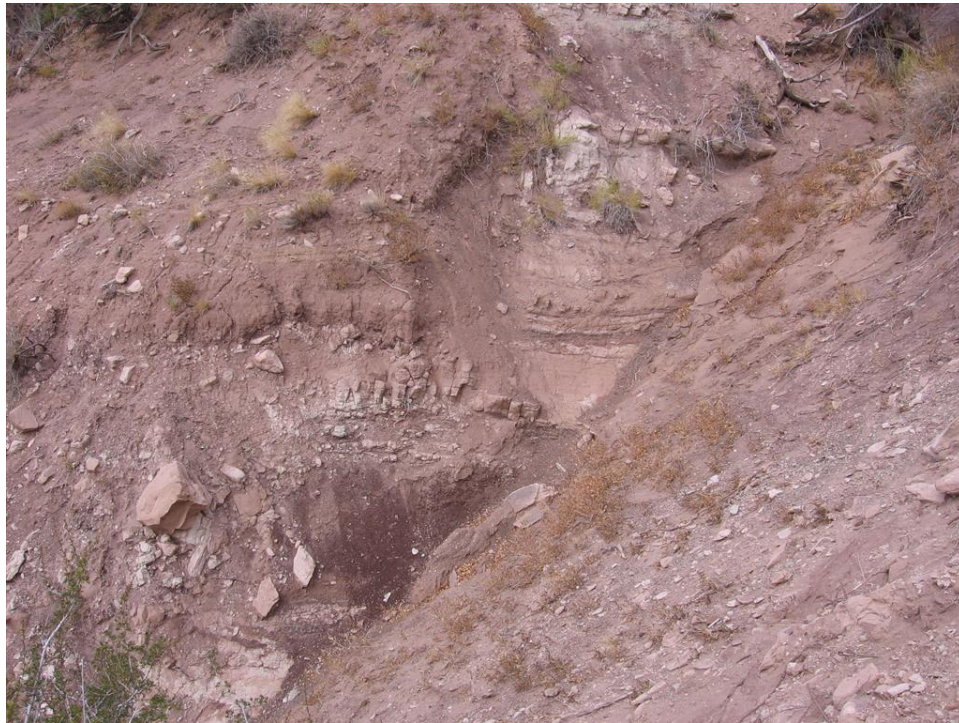
Photo 1. Walking pathway towards mine site washed out
