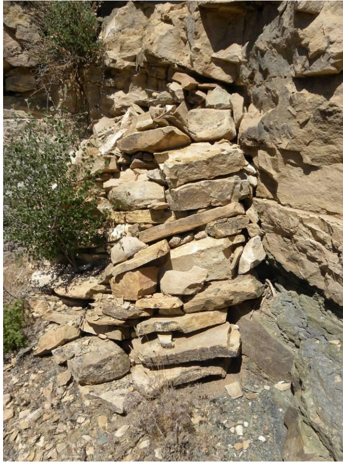
Photo 3. Adit with stone reclamation seal
