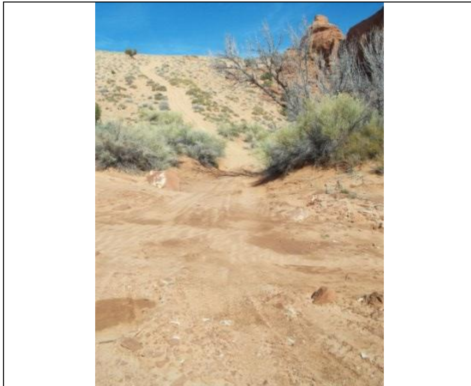
Photo 1 Impassable road in direction of the site
