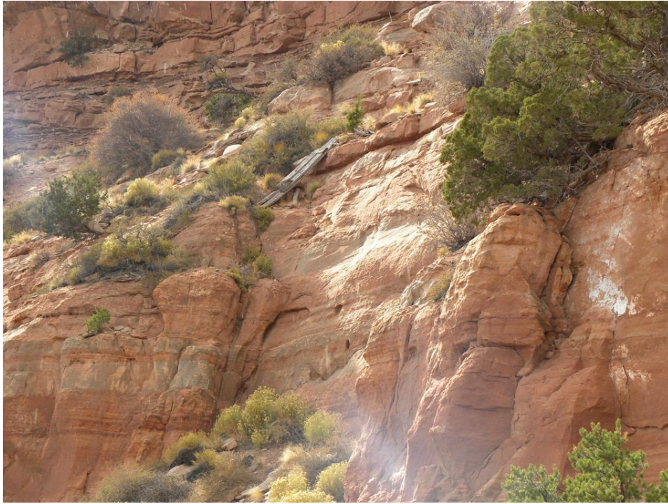
Photo 5. Wood debris along cliff face
