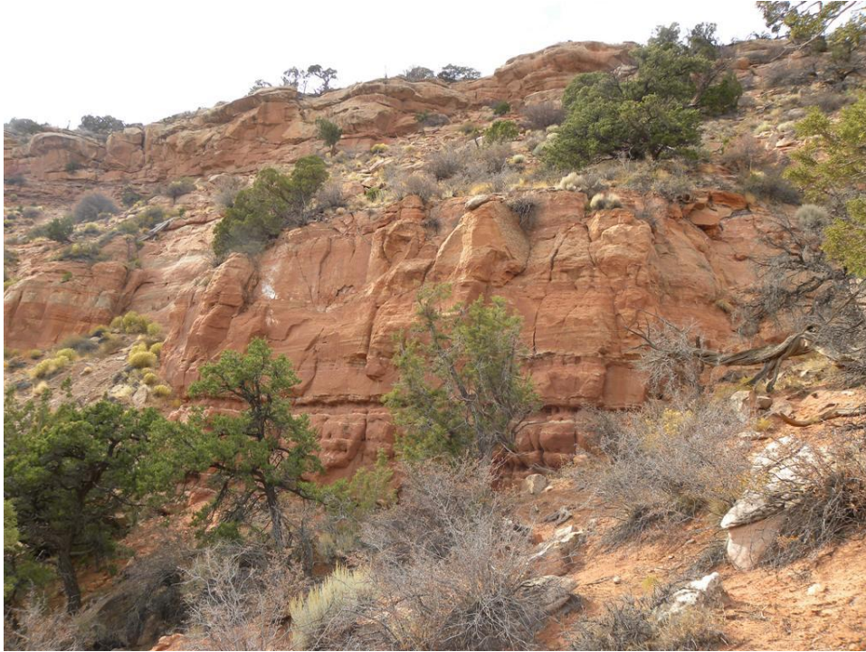
Photo 1. Cliff and debris area
