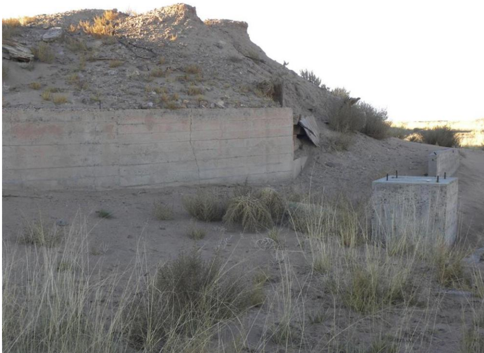
Photo 6. Section 9 Lease, Site #457, concrete structure area
