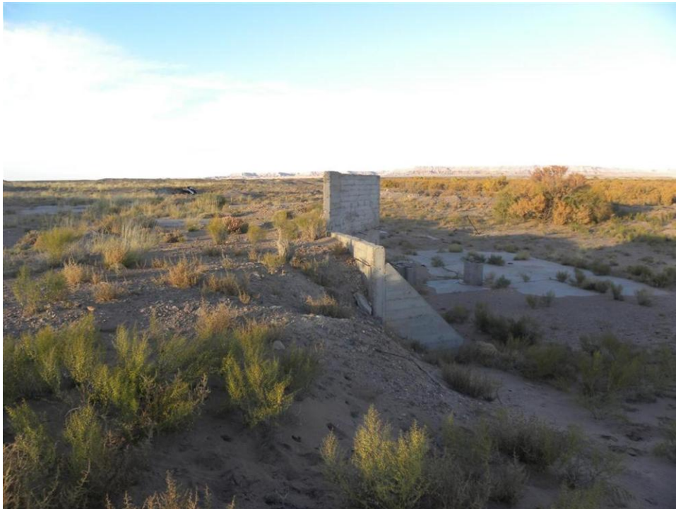
Photo 10. Section 9 Lease, Site #457, concrete structure area
