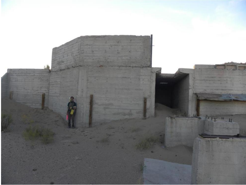
Photo 13. Section 9 Lease, Site #457, concrete structure area
