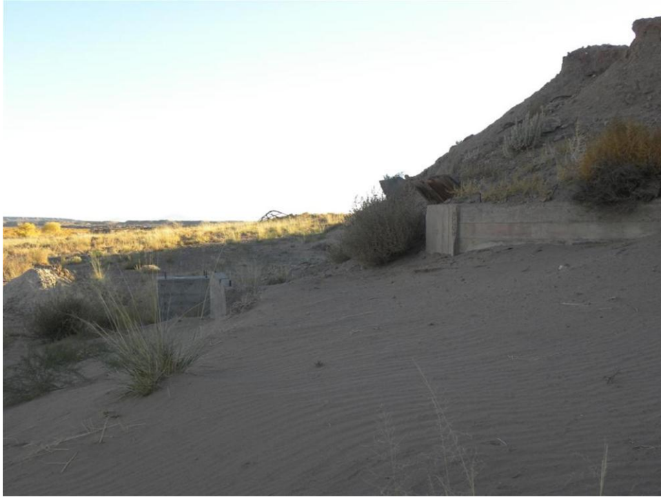
Photo 5. Section 9 Lease, Site #457, concrete structure area
