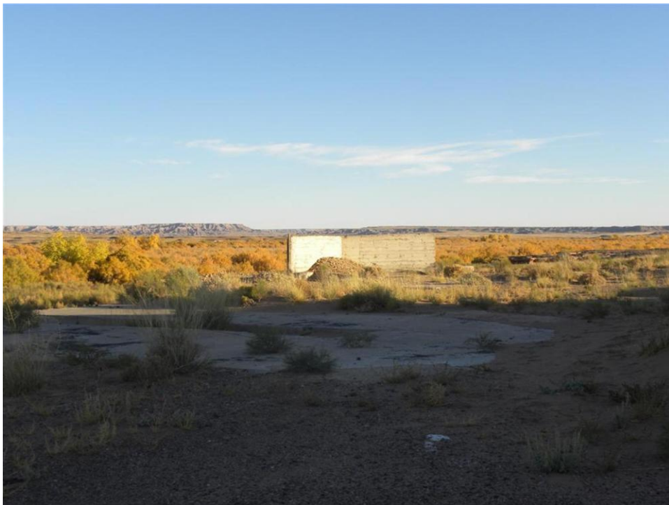
Photo 4. Section 9 Lease, Site #457, concrete structure area
