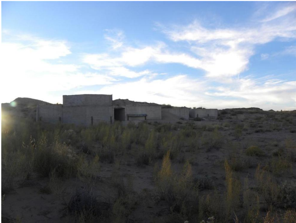
Photo 14. Section 9 Lease, Site #457, concrete structure area
