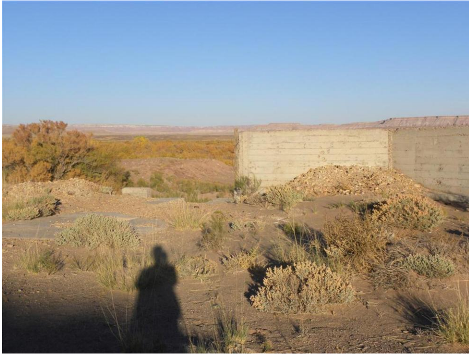
Photo 7. Section 9 Lease, Site #457, concrete structure area
