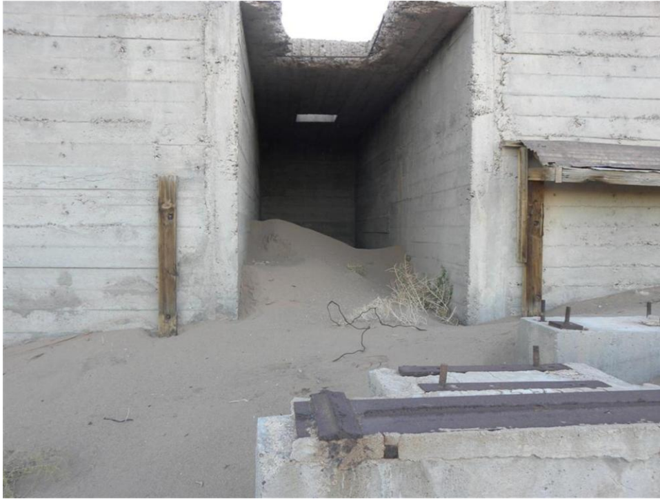
Photo 15. Section 9 Lease, Site #457, concrete structure area
