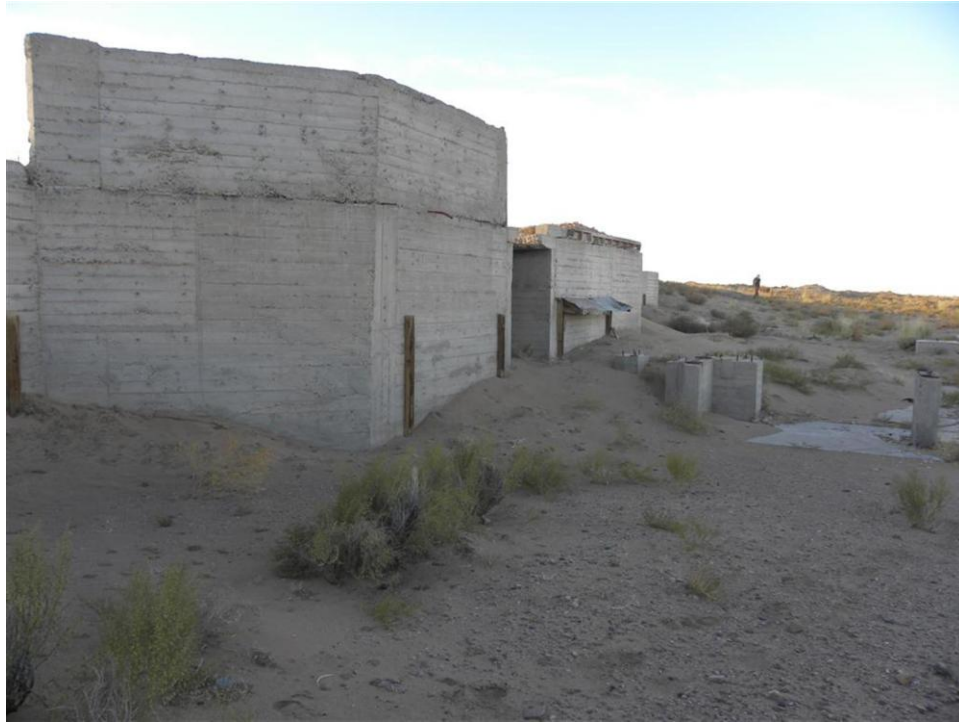
Photo 11. Section 9 Lease, Site #457, concrete structure area
