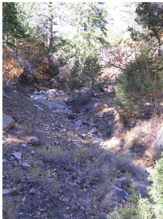
Photo 4. Drainage below concrete pad
