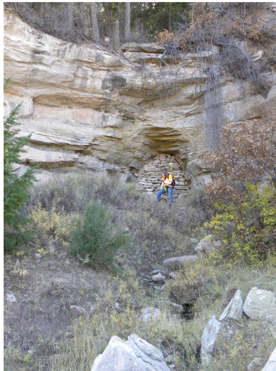
Photo 8. Sealed adit and drainage
