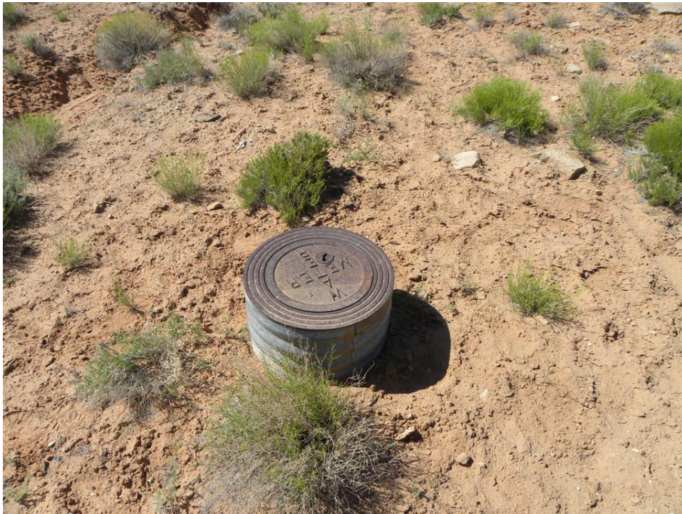
Photo 6, Plot 2 site, vent hole
