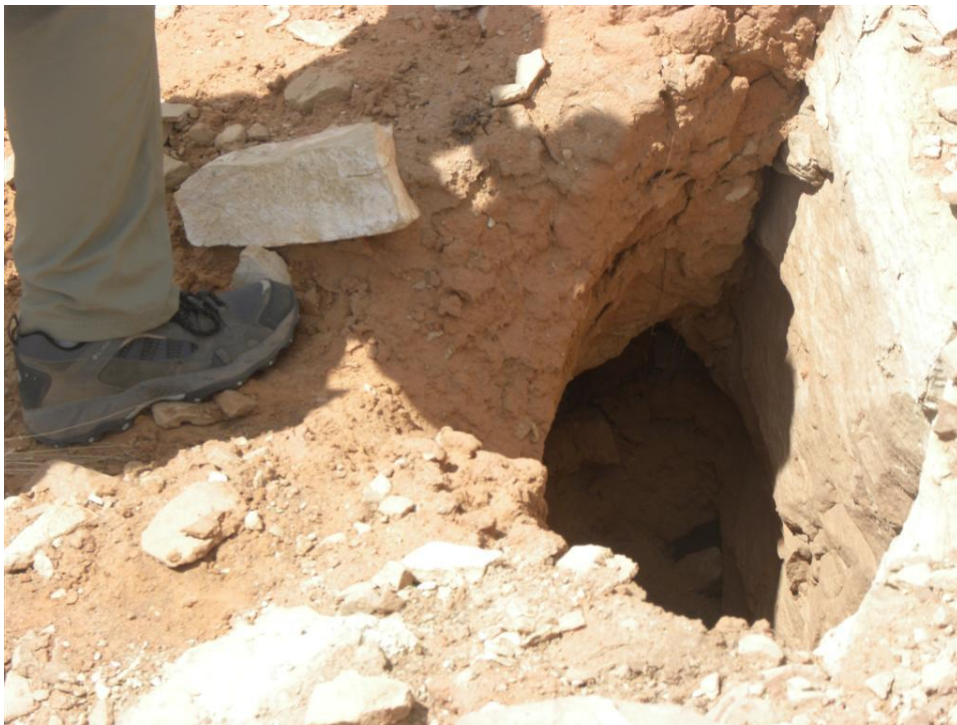
Photo 4. Black Rock Point Mines, hole above buried adit
