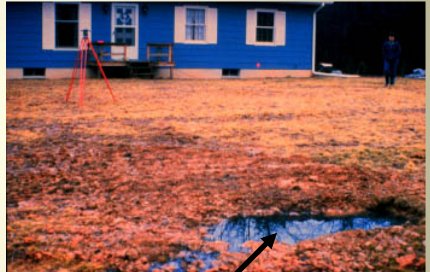
Sewage on the ground surface
