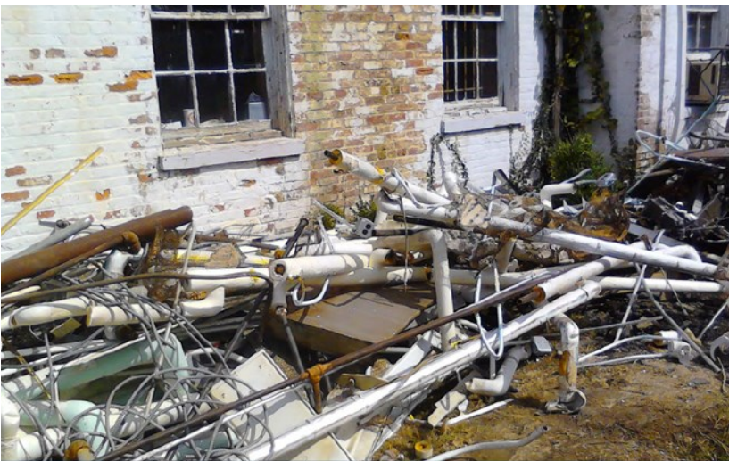
Asbestos-containing materials placed outside of building
