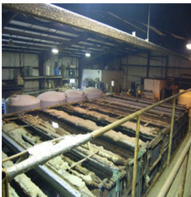
Inside Cedar Valley Electroplating facility
