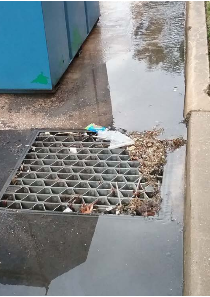
Ponding around the drain
