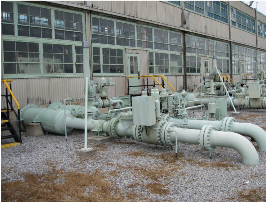
Rayne, LA: compressor unit valves (suction and discharge)
