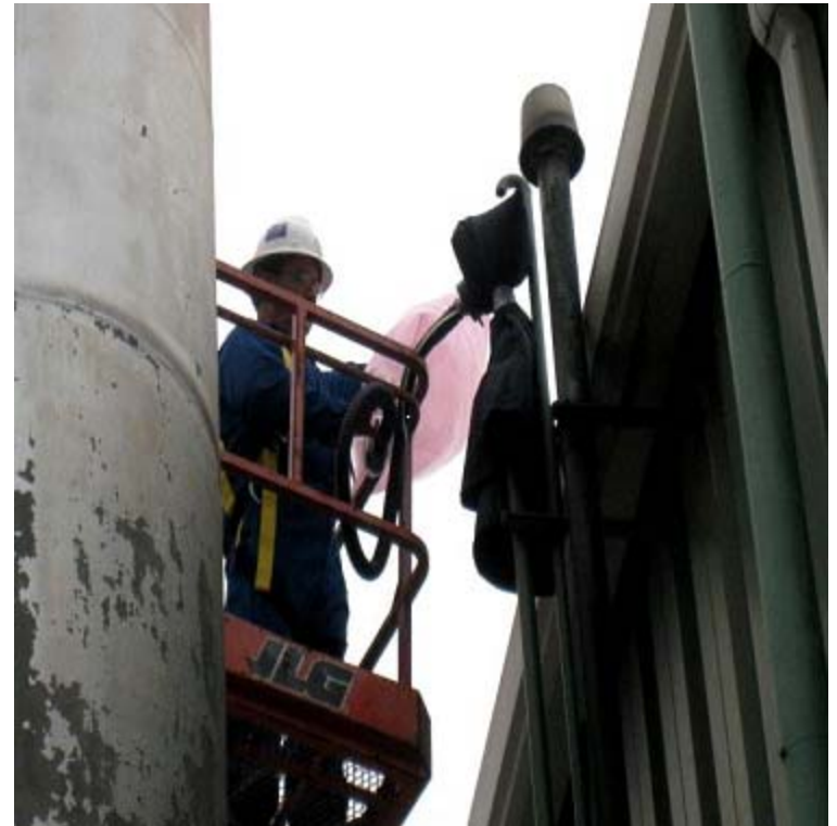
Using calibrated vent bag for rod packing emissions
