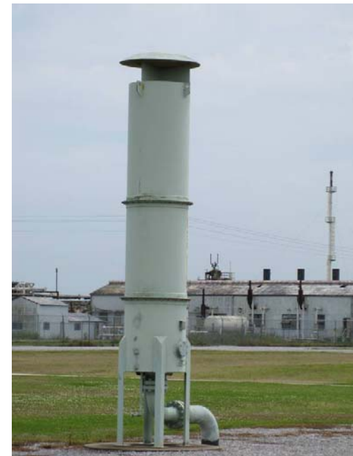
Rayne, LA: common blowdown vent
