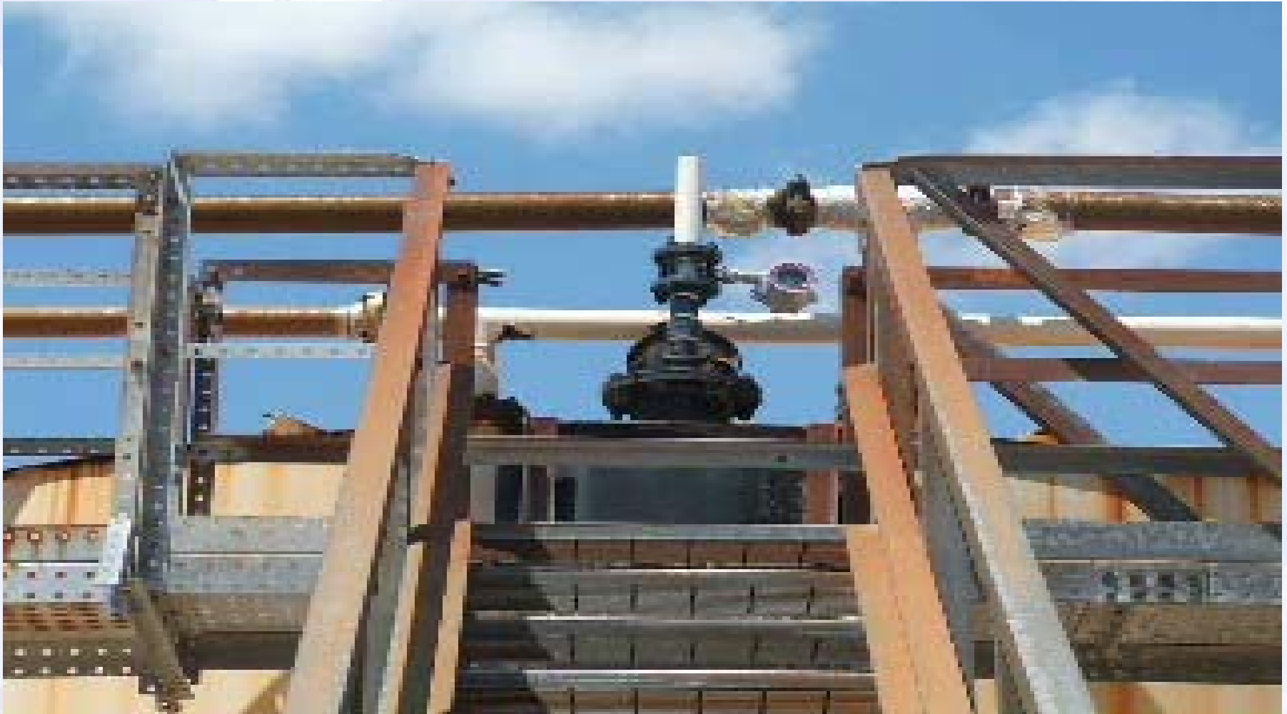
Example of Metering Equipment Installed in Thief Hatch
