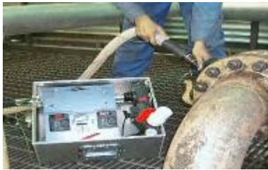
Oil and Gas Systems
