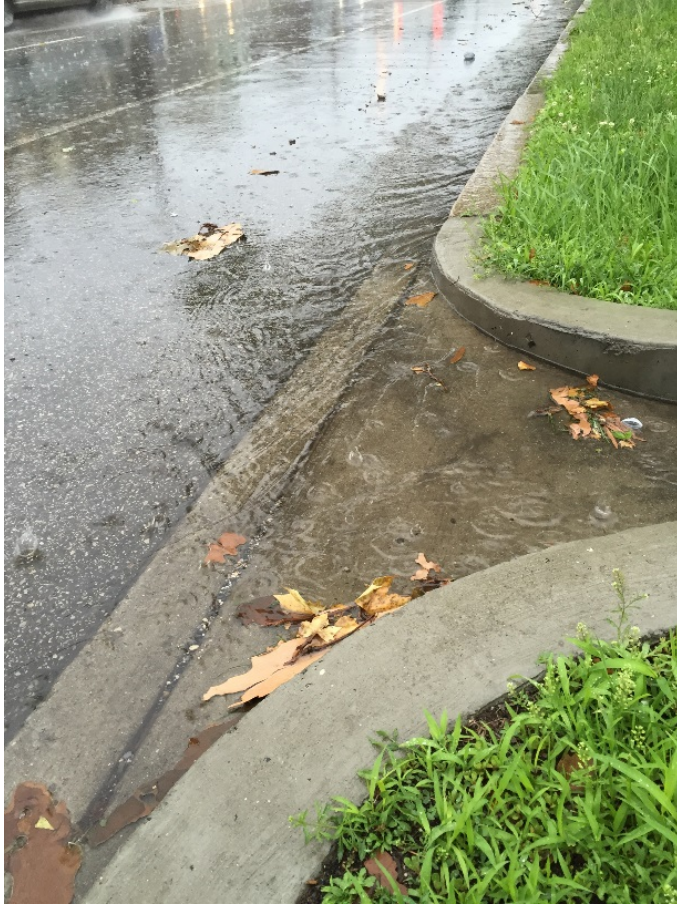
Surface flow bypassing trench drain
