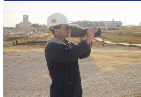
Infrared Leak Detection
