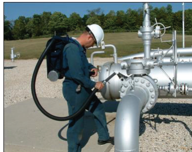
Leak Measurement Using High Volume Sampler
