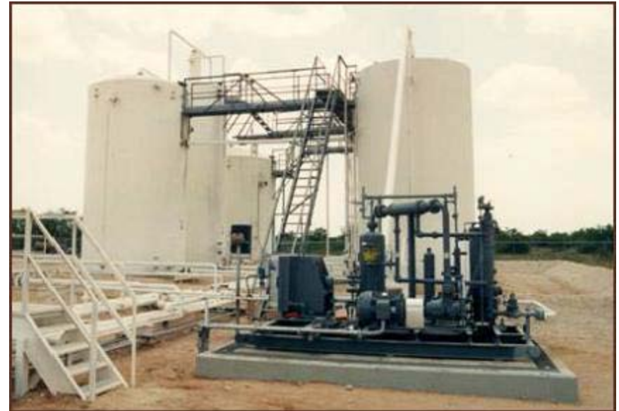
Source: Hy-Bon Engineering, VRU
