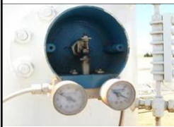
Invalco 415, 215, 402 Retrofit w/ Mizer valve, block & gauges
