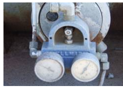
WellMark Flexlever This is the "old style" WellMark Replace/Retrofit with the entire Cemco head
