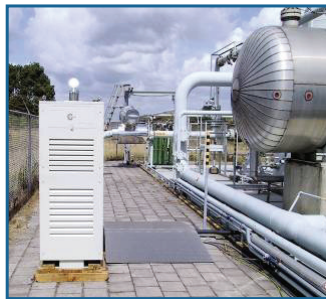
Test prior to platform deployment, Netherlands
