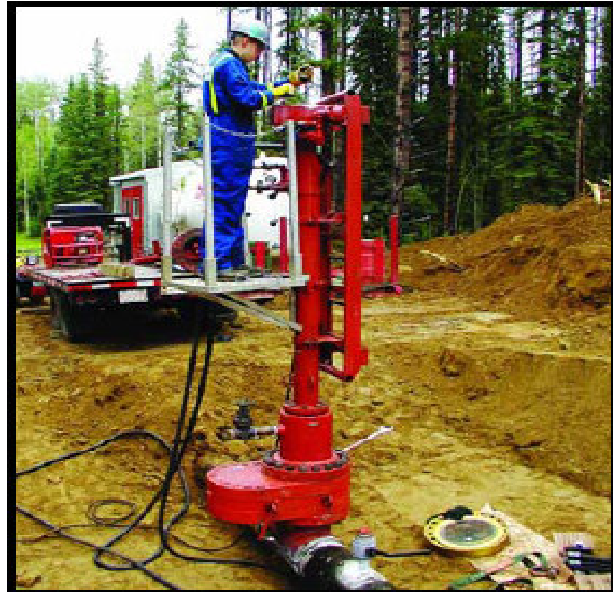
Certified Williamson Industries Technician performing a hot tap with a 760 Tapping Machine as part of a 12" Stopple application.
