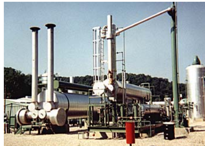
Glycol Dehydrator Unit Source: GasTech
