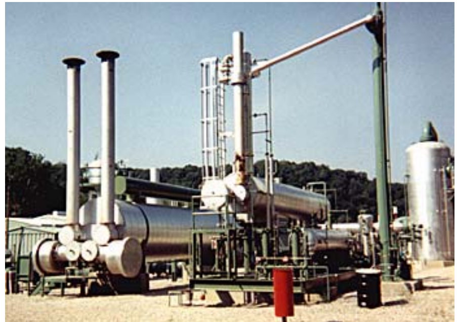
Glycol Dehydrator Unit Source: GasTech
