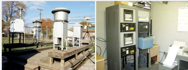
Typical Regulatory Monitors
