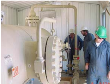
Three Phase Separator, Source: BP
